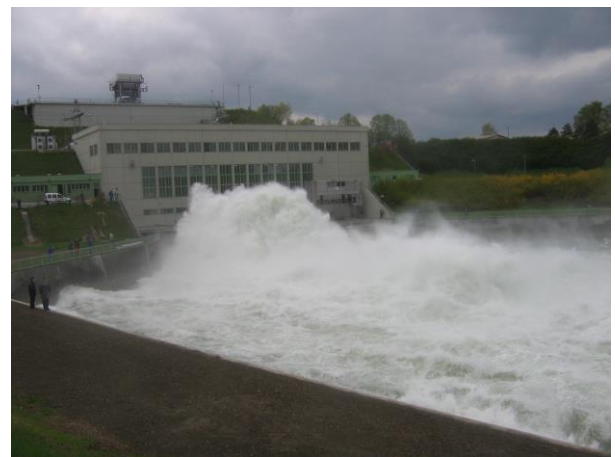
Fig.3: Action of pressure regulating valve during turbine shutdown in Zlatoličje HPP
