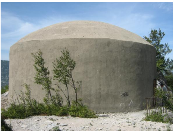
Fig. 5: Above-ground layout of the surge tank in Perućica HPP, Montenegro
