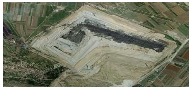
Fig.1: The open-pit coal mine "Drmno", Serbia
