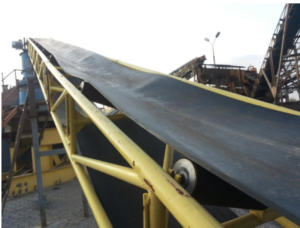
Fig.14: Belt conveyor after assembly
