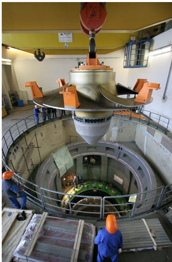
Fig.2: Lowering of 80 MW Kaplan runner in turbine pit; Zlatoličje HPP
